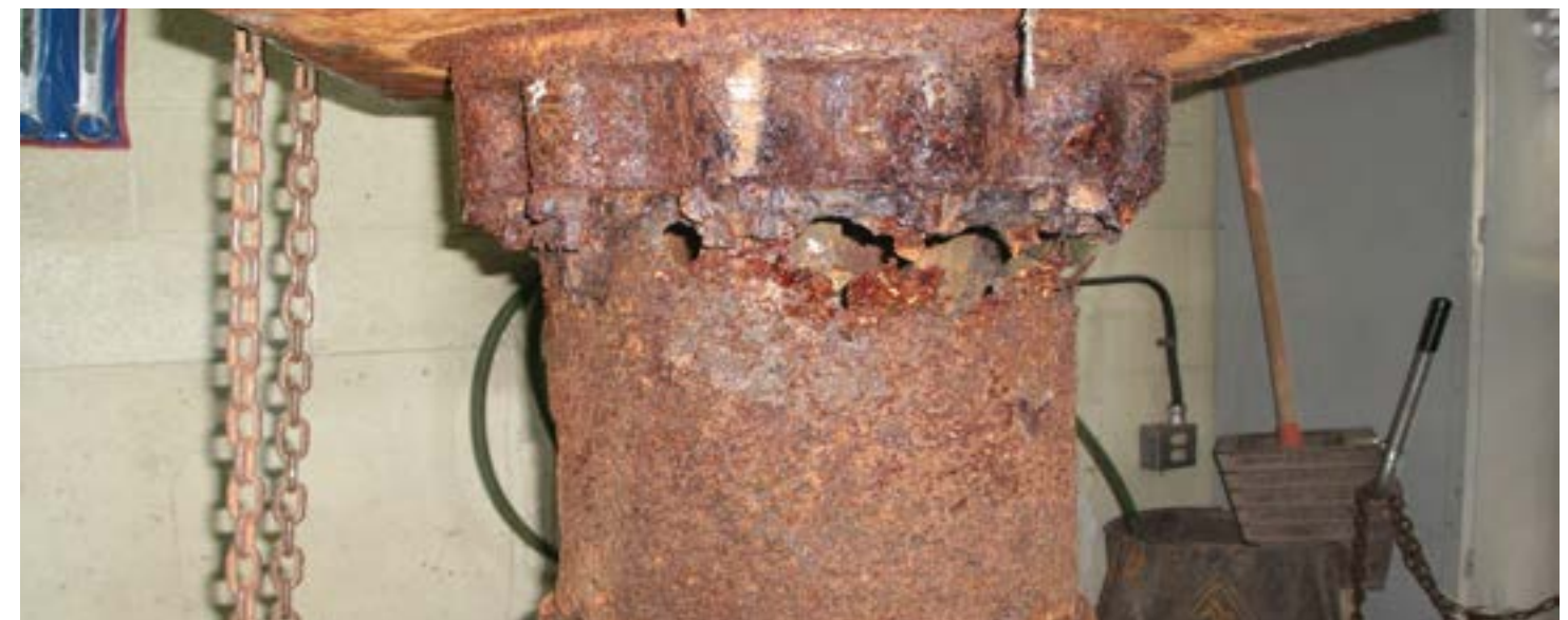
Partially corroded vertical turbine pump column attached to the discharge head. Pump still functioned at a lower efficiency of course!
